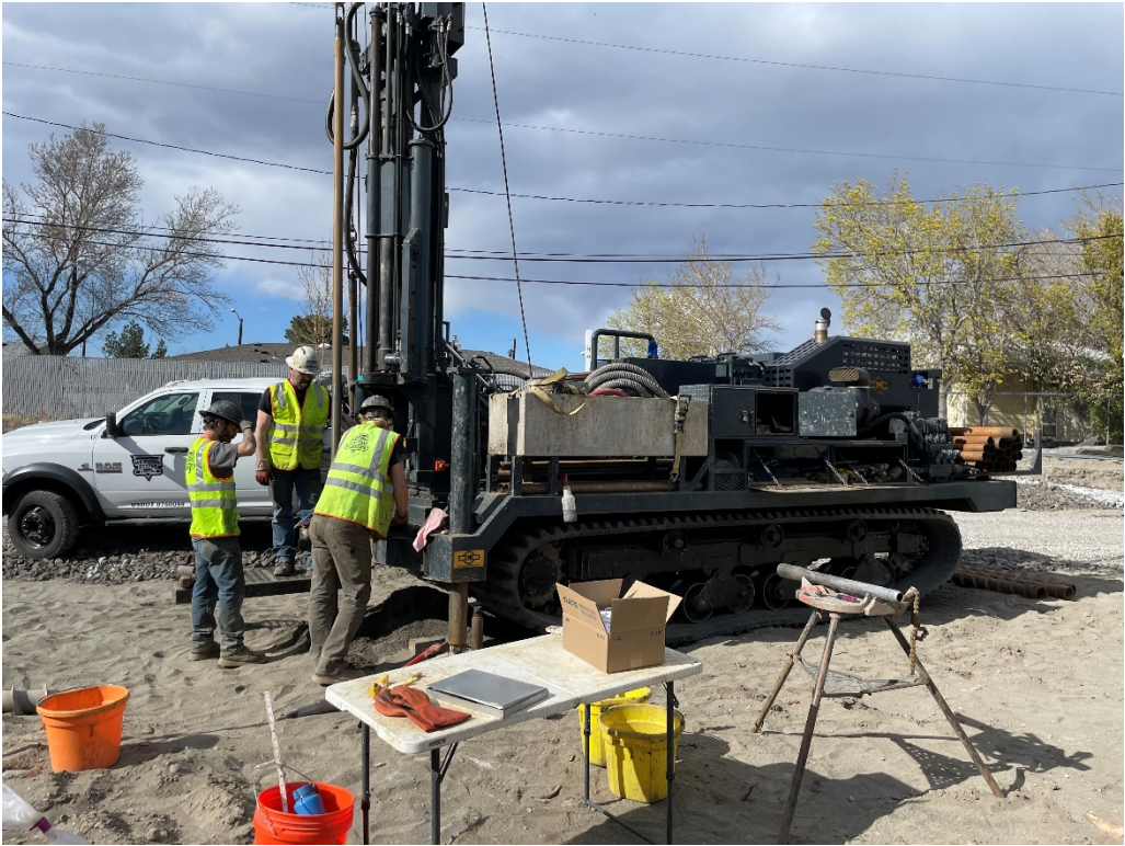
Exhibit 3 - Showing a typical drill site with the tracked rig, and support truck.
